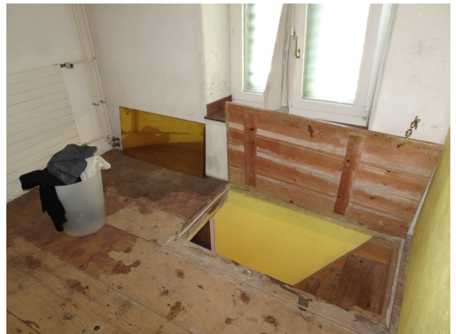
EG ex 29 Waschen UG-Treppe west
